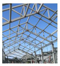
The Hotel's structure is framed entirely in galvanized light gauge steel providing two design functions, a non-combustible rating, and a durable building material necessary in coastal projects. The total construction cost was approximately \$30 million.
